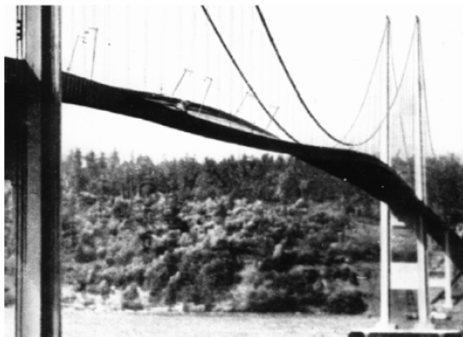
Tacoma Narrows Bridge Collapse, 1940 Source: Münchner Rück (1990)
